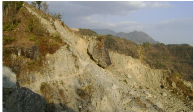
2. Landslide at Ramche
